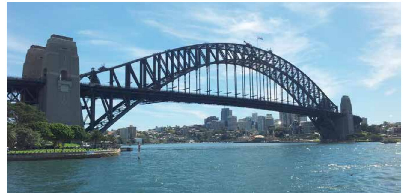
The Sydney Harbour Bridge connects the CBD with the North Shore and is popular for walks, bridge climbs, tourists as well as being an integral part of Sydney's New Year's Eve celebrations.
