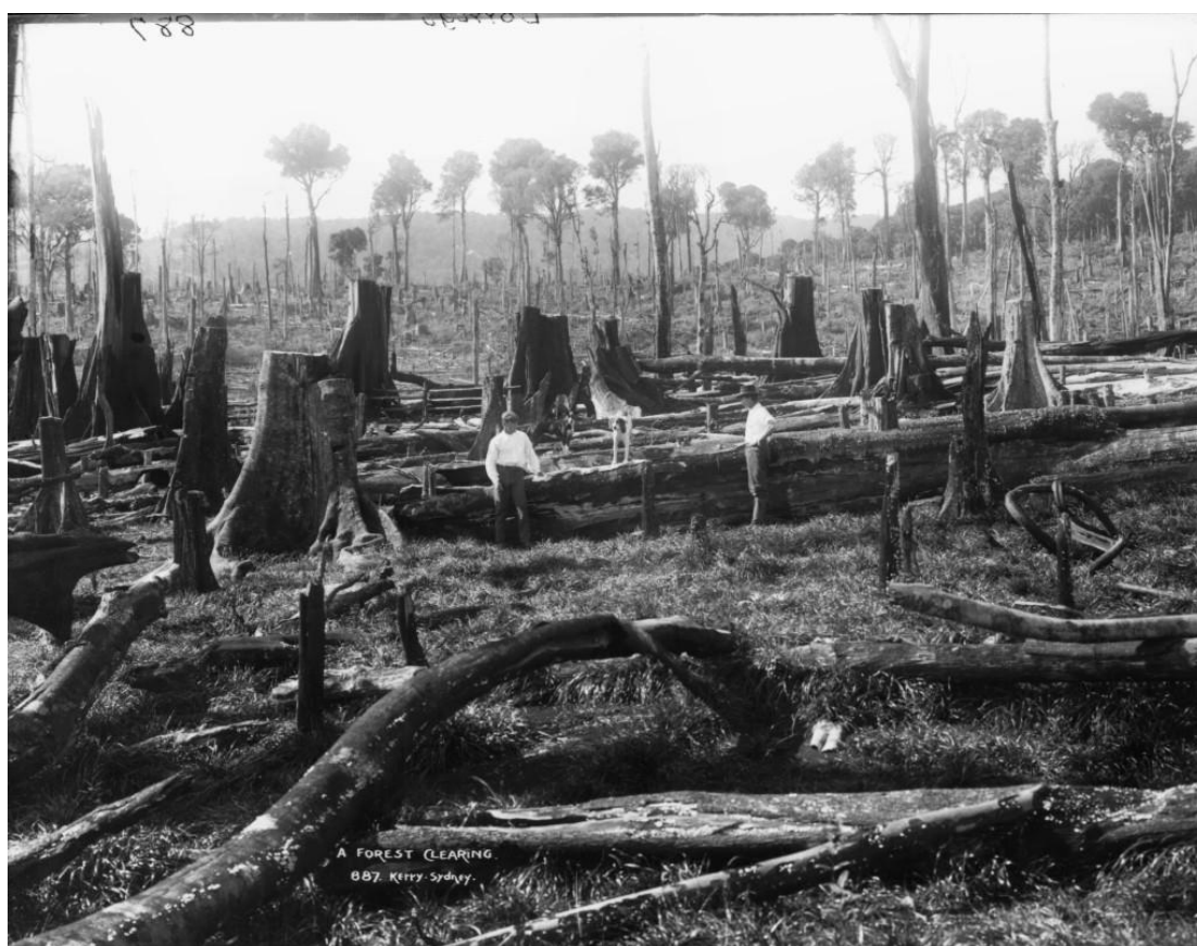
Figure 4.16 Forest clearing in Sydney Harbour catchment (Kerry and Co, 1905)
