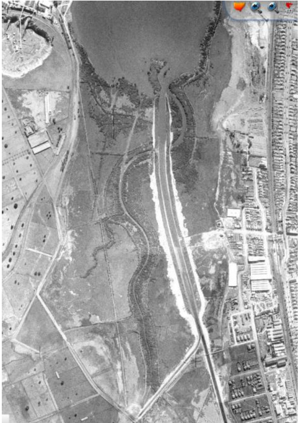
Figure 4.5 Homebush Bay in 1943 showing the newly constructed stormwater channel cut through the original meandering course of Powells Creek (image from SIX Maps, NSW Department of Finance, Services and Innovation).
